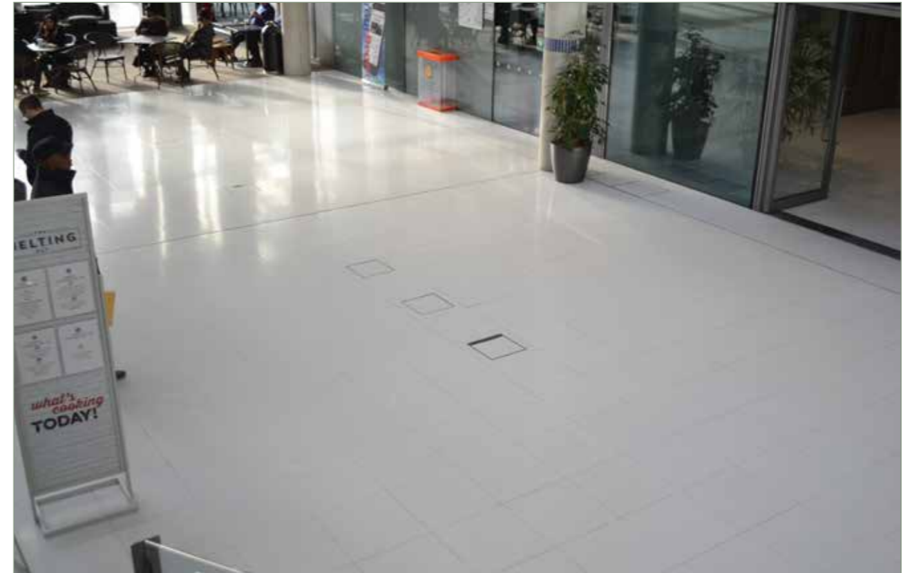
This box is used where depth restrictions are in place. Removing the RCBO protection and the use of tiles instead of pavers facilitates the shallow 225mm depth.
