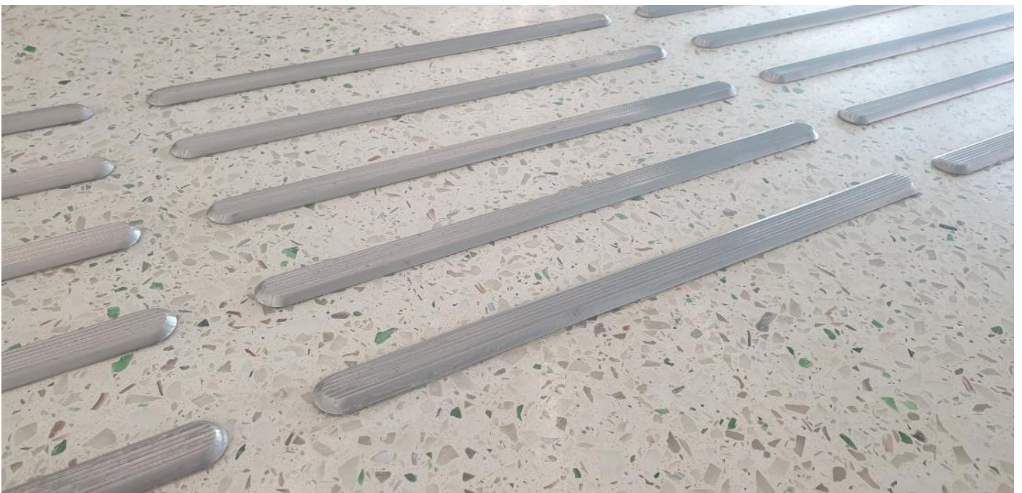
Typical array of Kent Ridge Tactile Warning Strips
